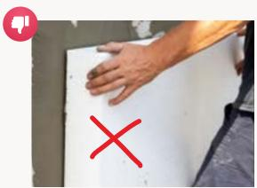
Avoid expanded foam (e.g., expanded polystyrene) insulation
