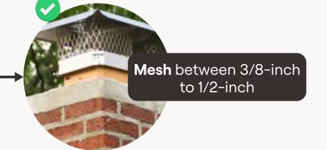
This mesh is **coarser** than what is used elsewhere to protect against embers (meaning it offers less protection against them) to ensure proper ventilation from your fireplace. Close damper during fire weather or after each use to protect against ember entry.
